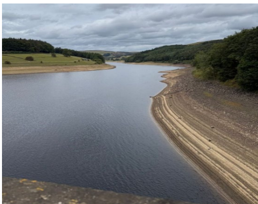
Figure 4: "Ladybower dam. Low water levels."
